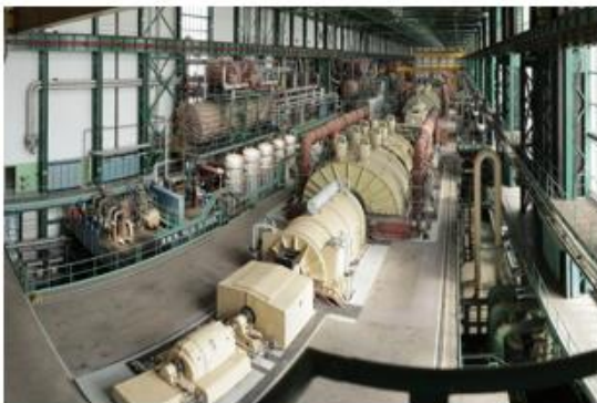
Turbine hall before any dismantling (05/2013)
