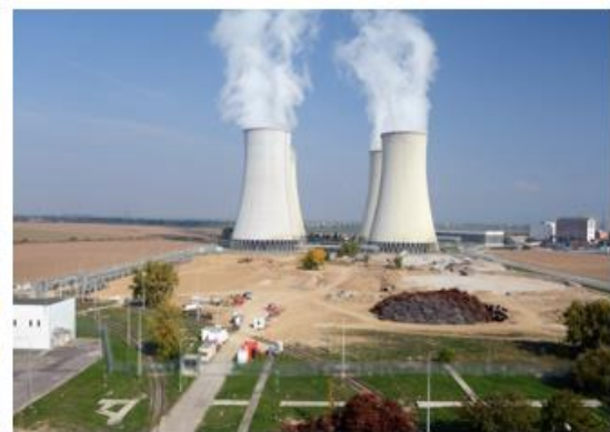
After demolition of 4 cooling towers (10/2018)
