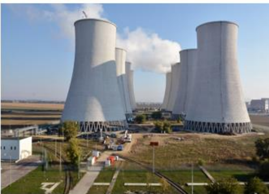
Before demolition of 4 cooling towers (09/2017)
