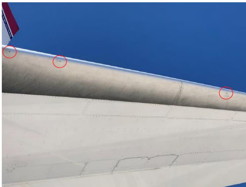
Picture 8: aircraft damage, horizontal stabilizer.
